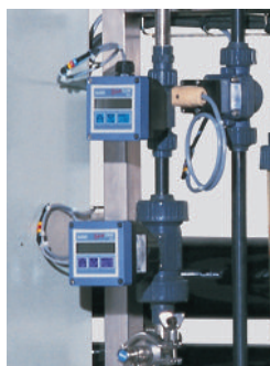
Analog sensor of loop flow rate and bacteriological sampling.
