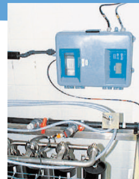
Ongoing supervision and analysis of the total and free chlorine.
