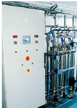
Septon Electrodesionisation, Clinique Cabestany.
