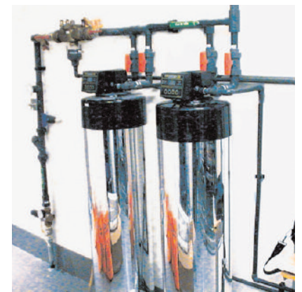
Sand pre-filtration for heavily loaded water.
