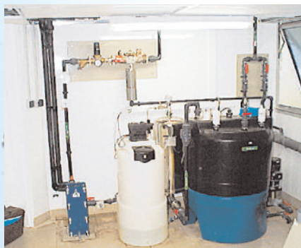
Cooling and pressurizing of tap water.
