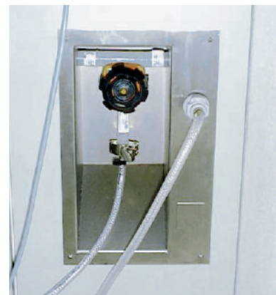
Sanitary « pharma » valve in PVDF or stainless steel with no dead legs.
