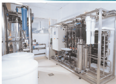
Compact water treatment system for autodialysis unit. Pure steam generator
