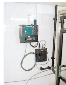
Ongoing supervision and analysis of the total and free chlorine.
