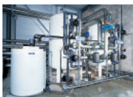
Clarification unit for river water. Automatic air / water wash filters
