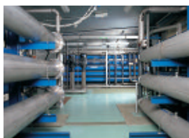
3 reverse osmosis units, 1 x 50 m 3 / hr and 2 x 35 m 3 / hr.
