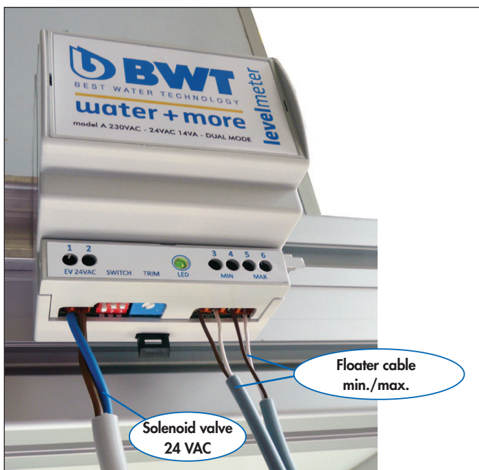
Fig. 6: Connection of the control cable (2-pin plug connection)
